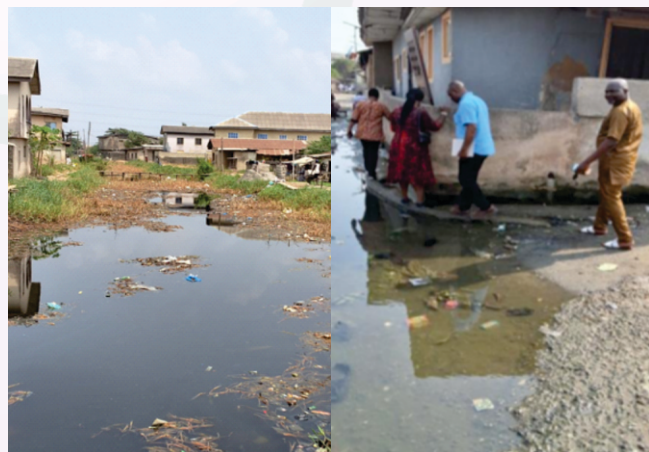
Plate 5: Image of Flood water on the road and a blocked drainage in Ijora Community Source: Palm-Trees Field work, February 2025.
